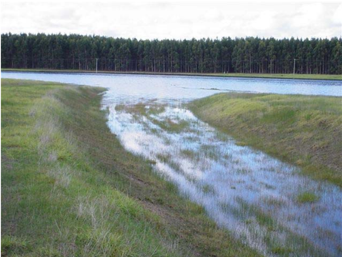
Photo 4 Main irrigation storage dam at commencement of overflow, July 2005
