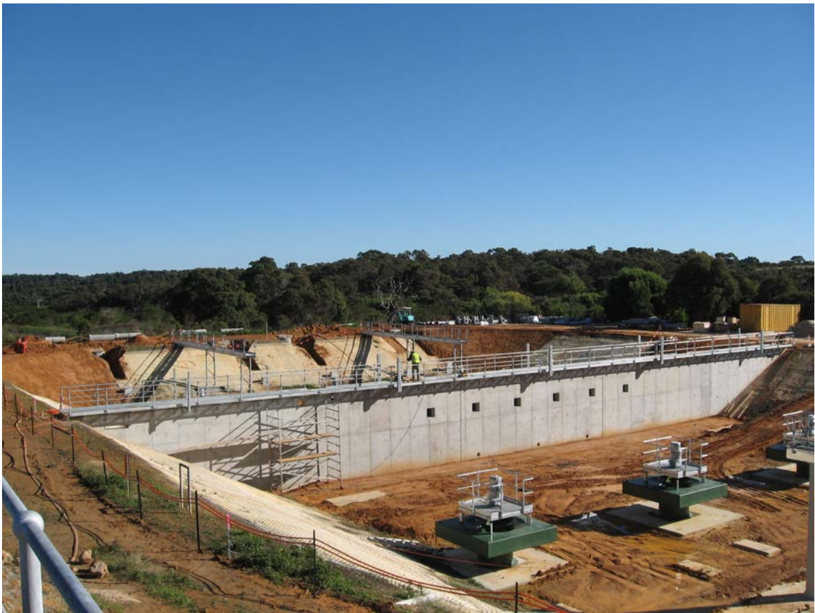
Photo 6 Timewell Road WWTP upgrade works, June 2006
