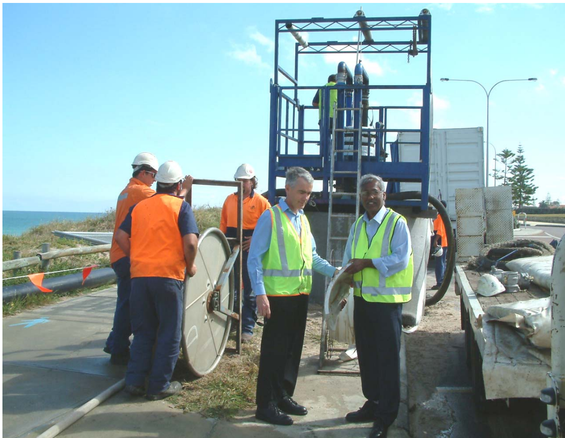
Improving Perth's wastewater system: Trenchless sewer relining project in Cottesloe
