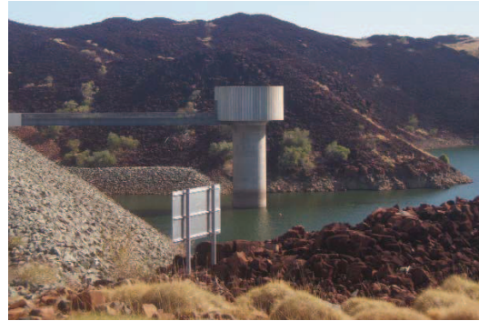
The West Pilbara water supply scheme draws water from the Harding Dam (pictured) and the Millstream Aquifer
