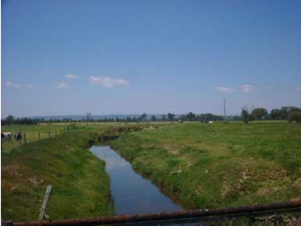
Photograph 5 Medium sized drain within private property
