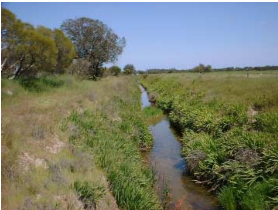
Photograph 4 Medium sized drain within a drain reserve
