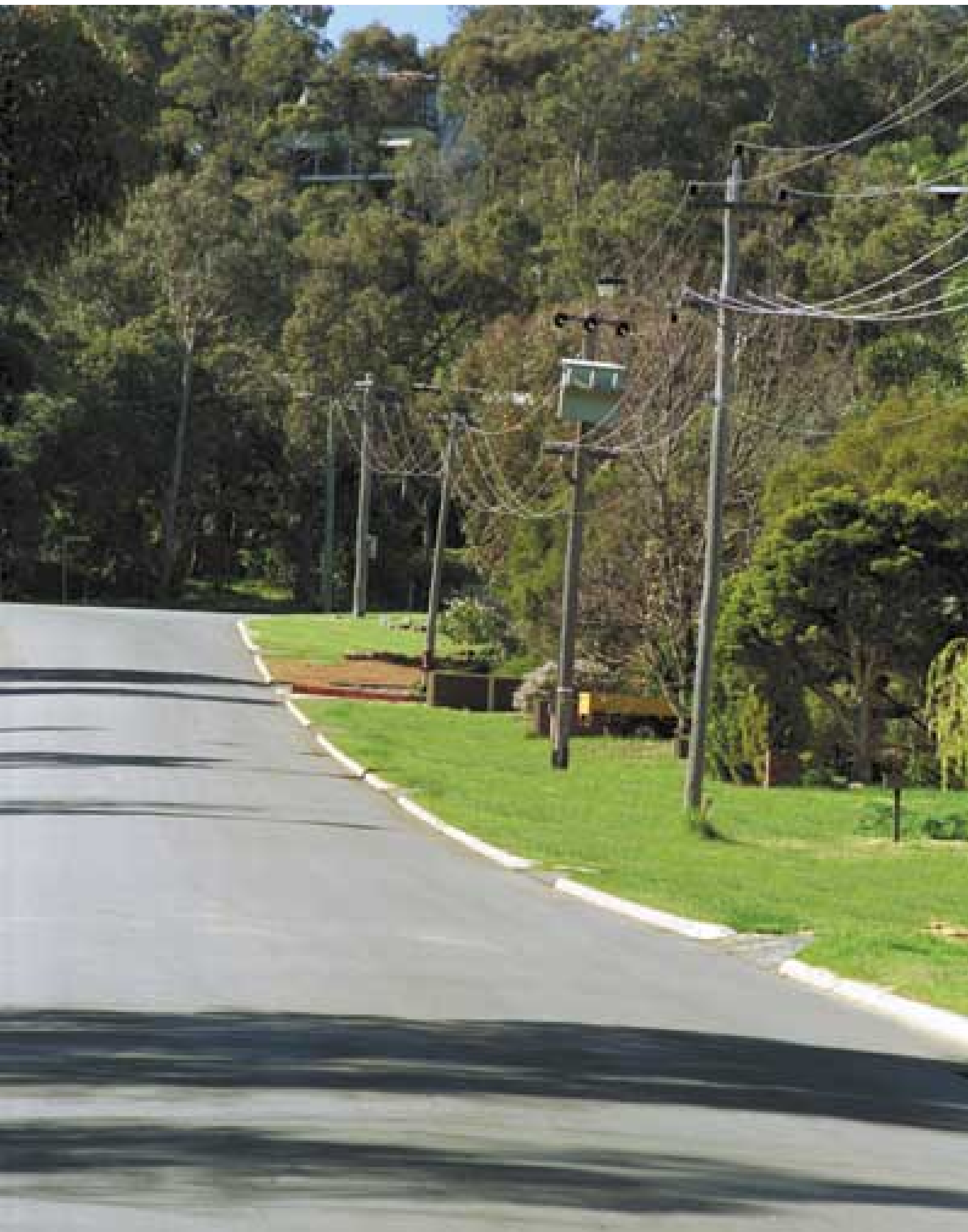
A Kelmscott street after infill sewerage work was completed.
