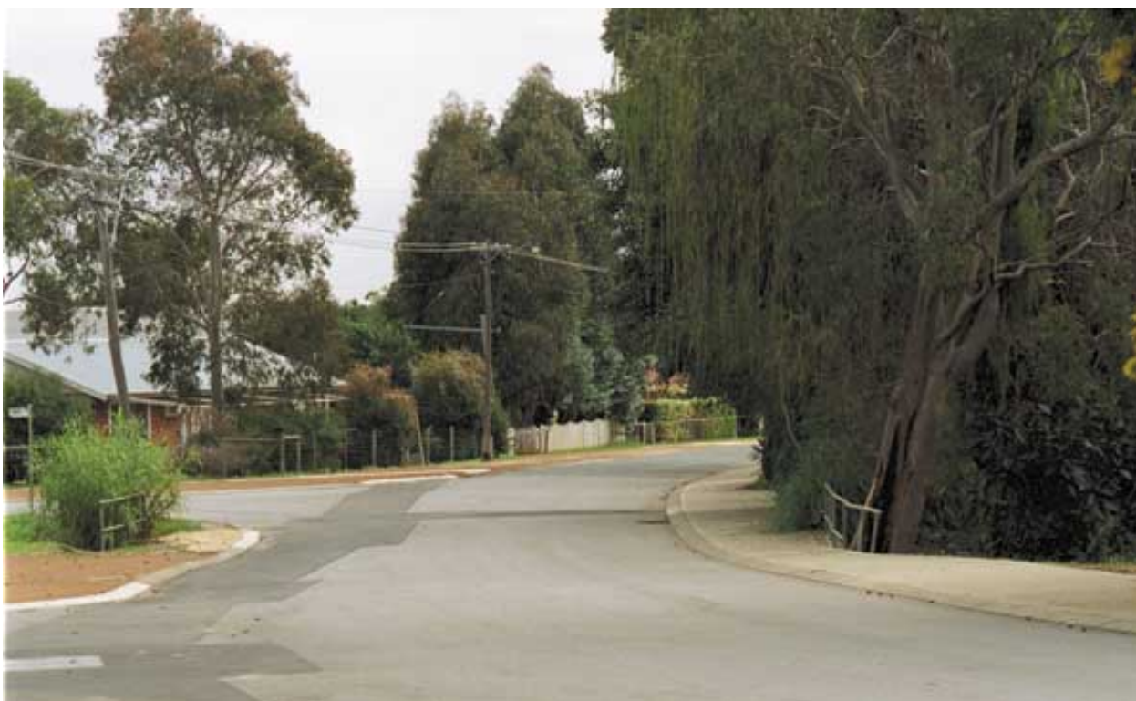
A typical street in Byford after infill sewerage work was completed.
